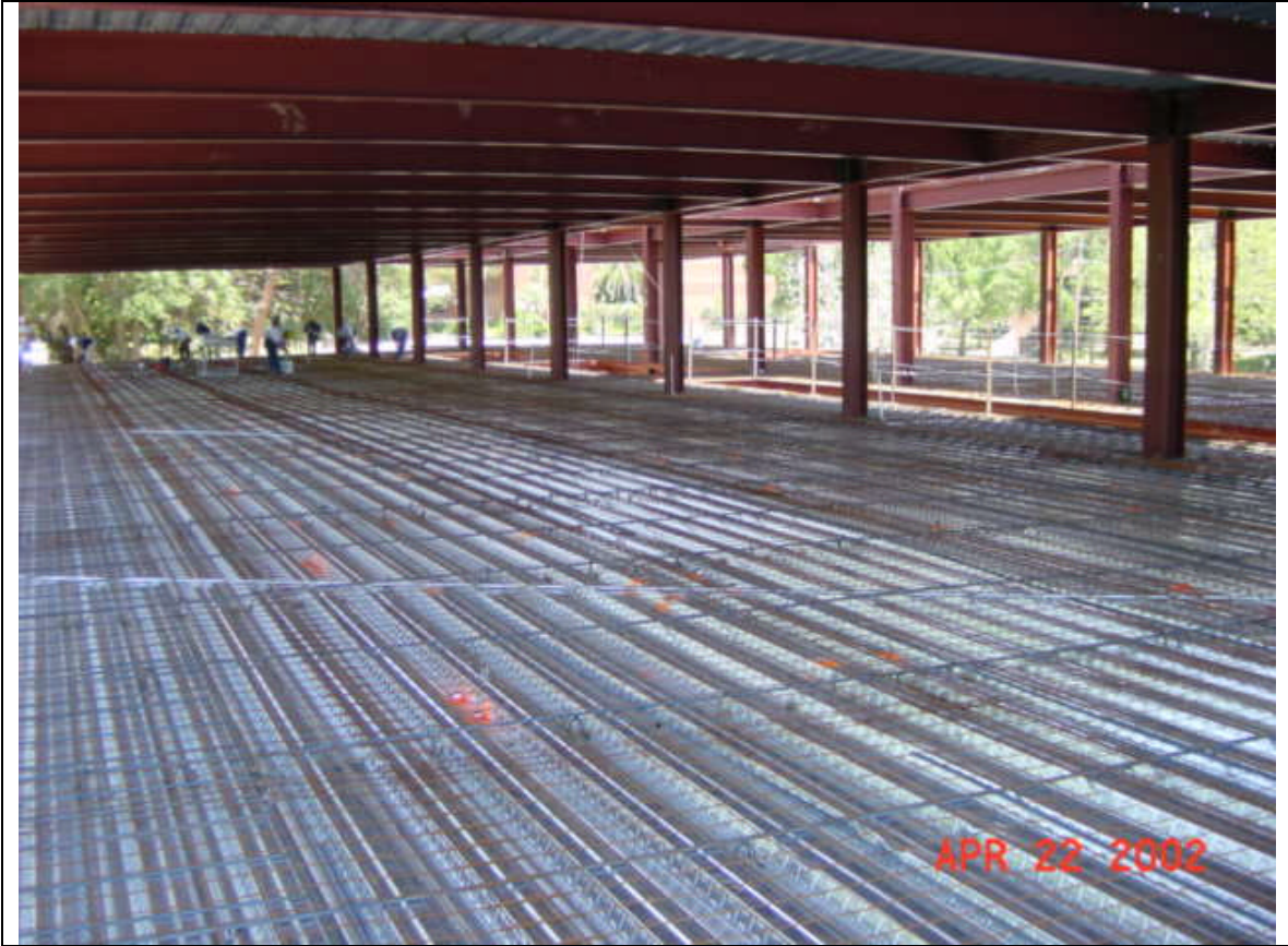
2nd Floor Prior to Pour.JPG
