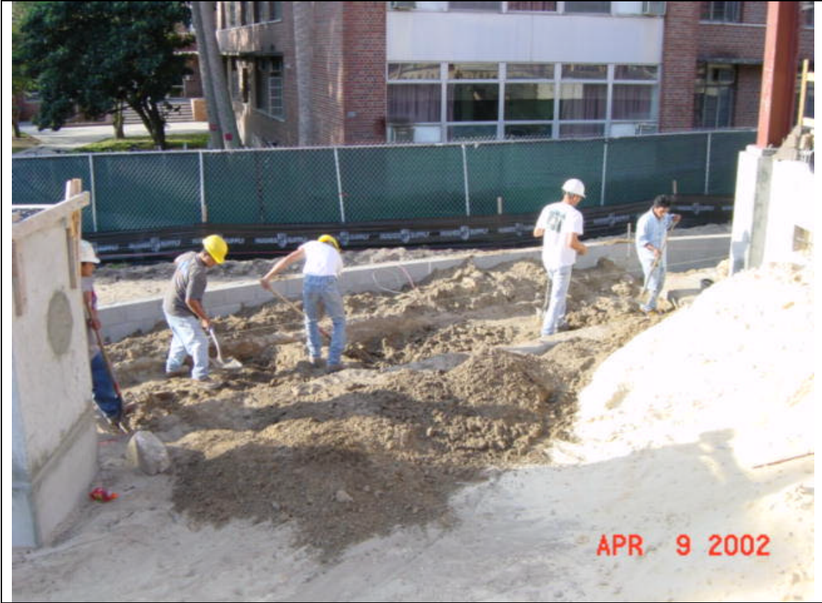
Excavation for Const. Yard Fnd...JPG
