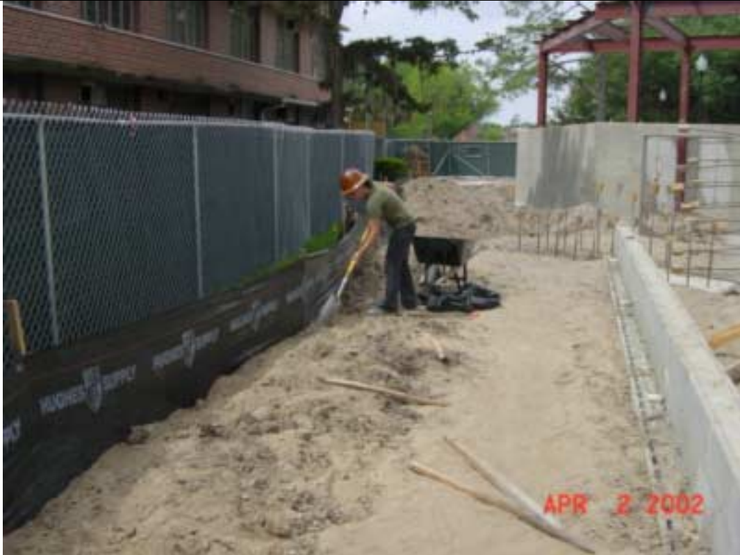
Maintenance of Silt Fence.JPG
