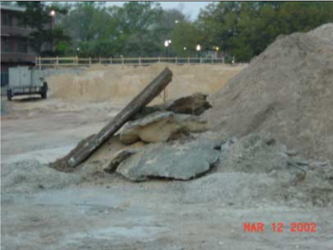
:Concrete and CMU stored for recycling.JPG
