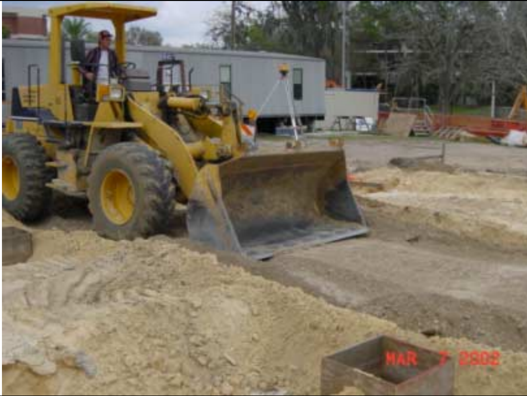
Salvaged Limerock used as crane road.JPG
