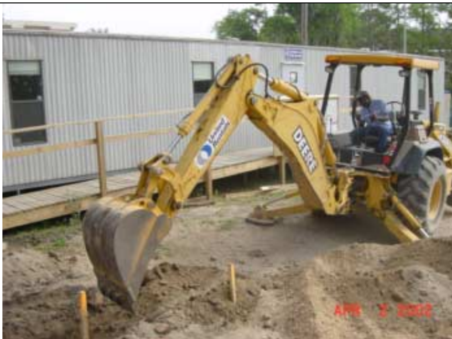
Excavating Revised A2 pad.JPG
