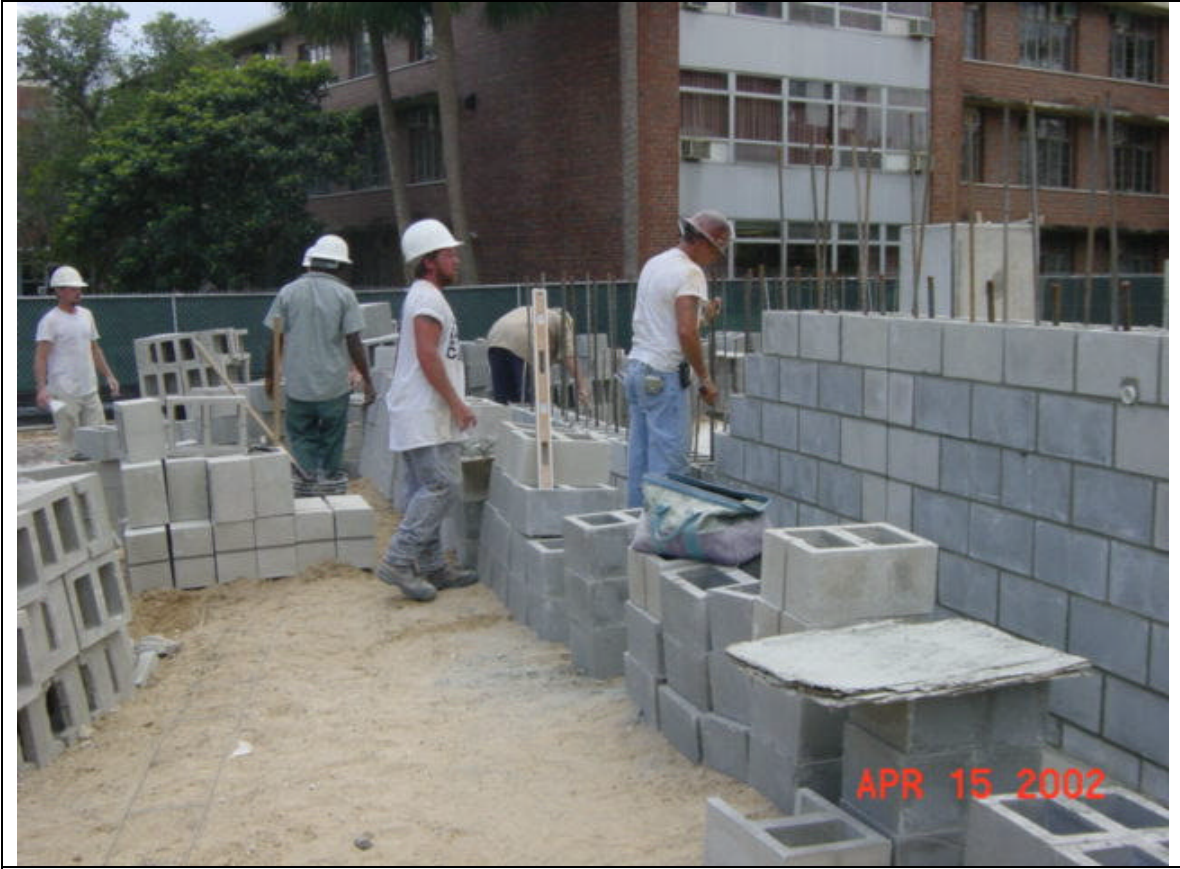
Construction yard wall.JPG
