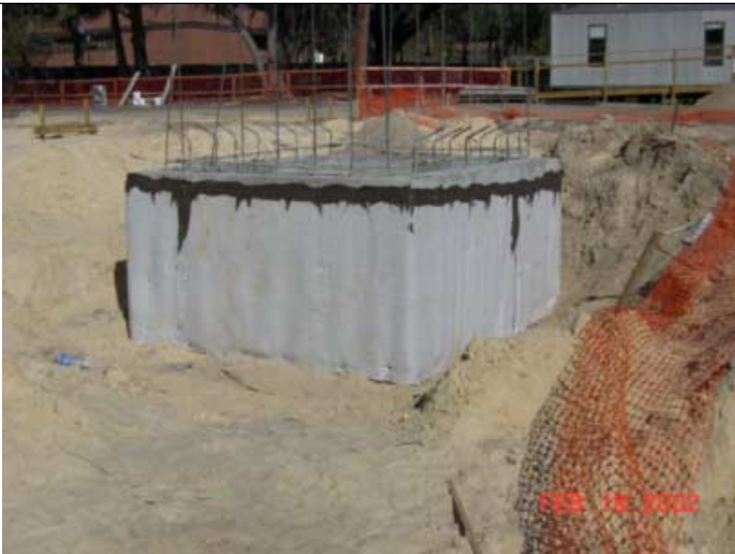
Elevator pit walls
