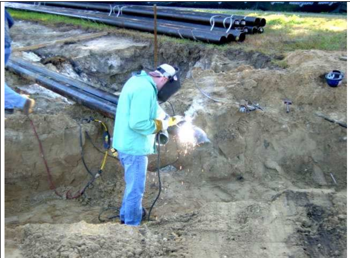
Welding chilled water pipes.
