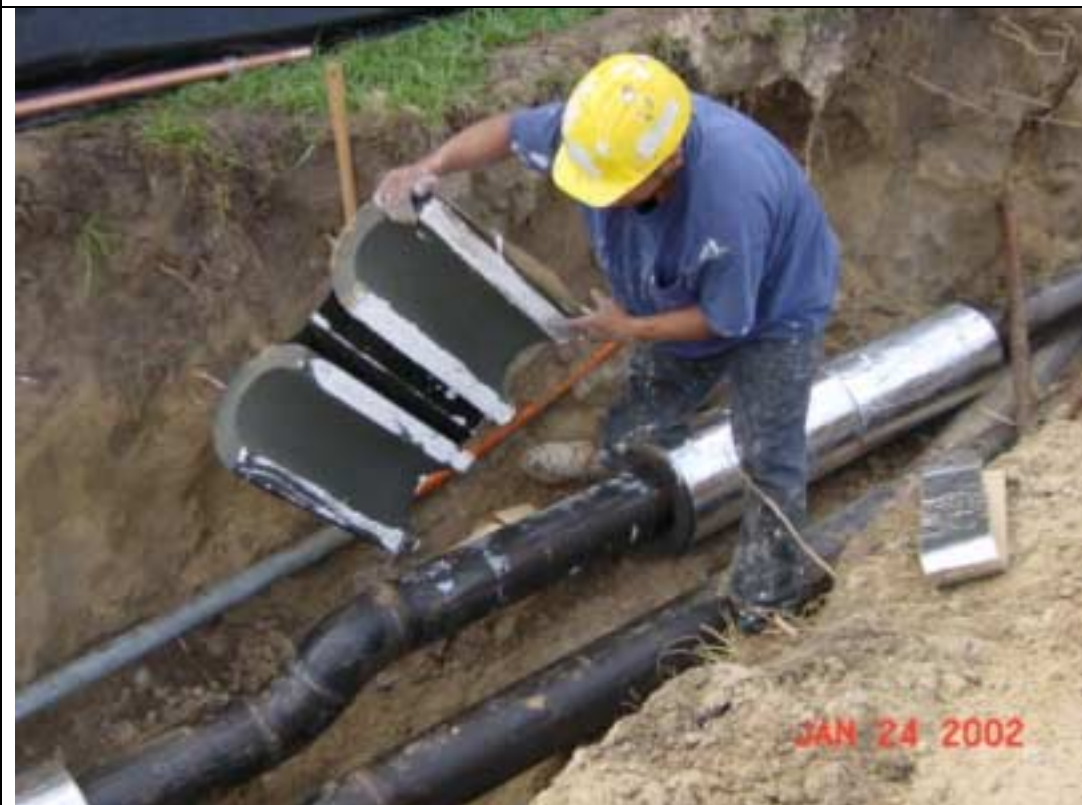
Insulating the chilled water line.
