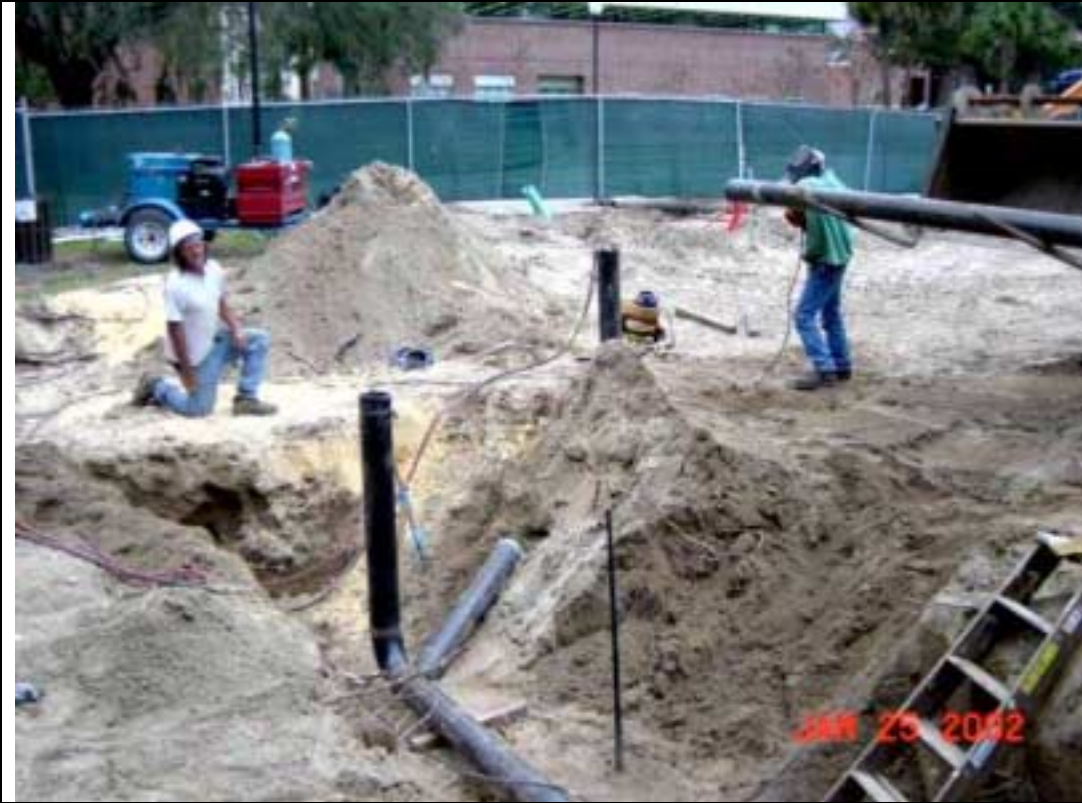
Chilled water line being stubbed into the building.
