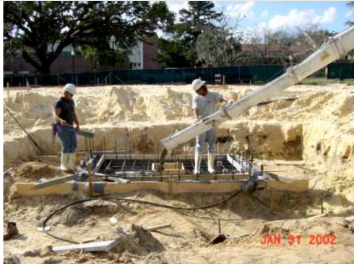
Placing concrete for the elevator pit.
