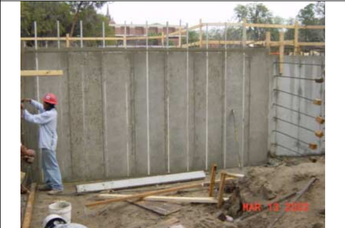
Dovetail Slots for Brick
