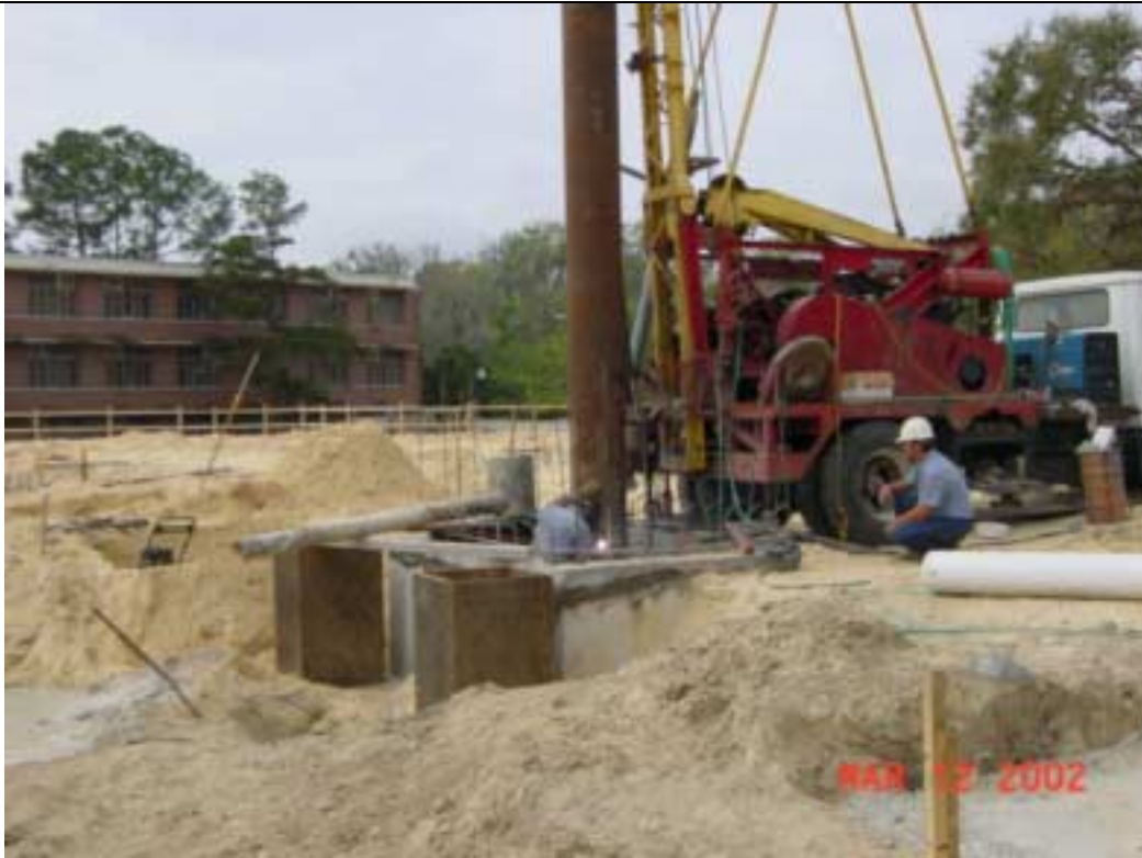
Drill Rig in Action
