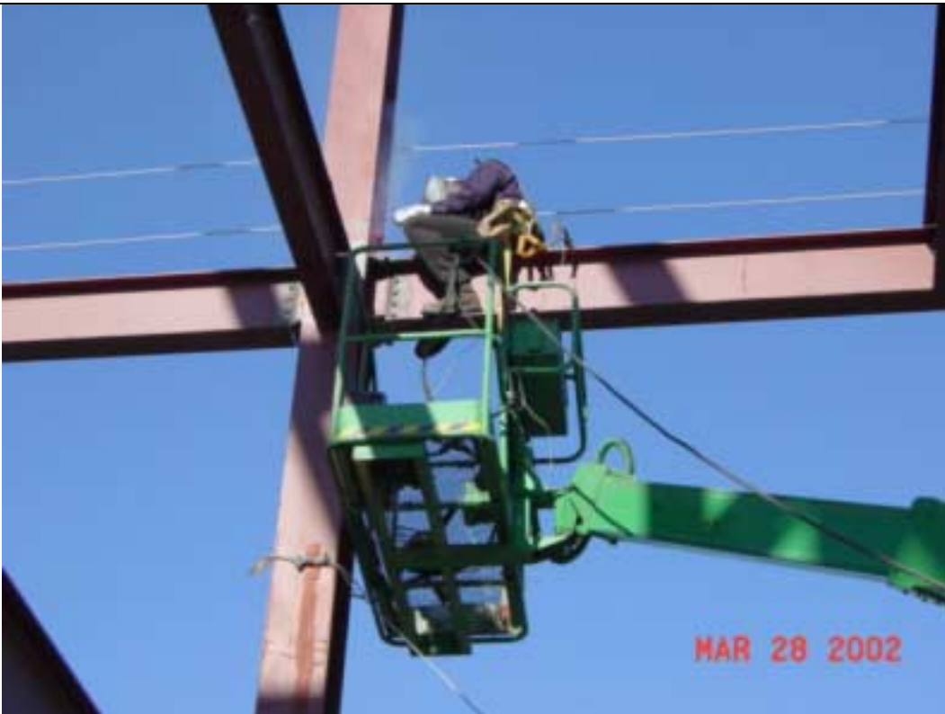
Welding at Moment connection.JPG
