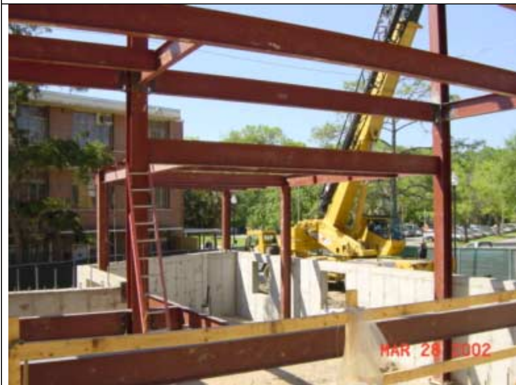
Mech. Room Roof Framing.JPG
