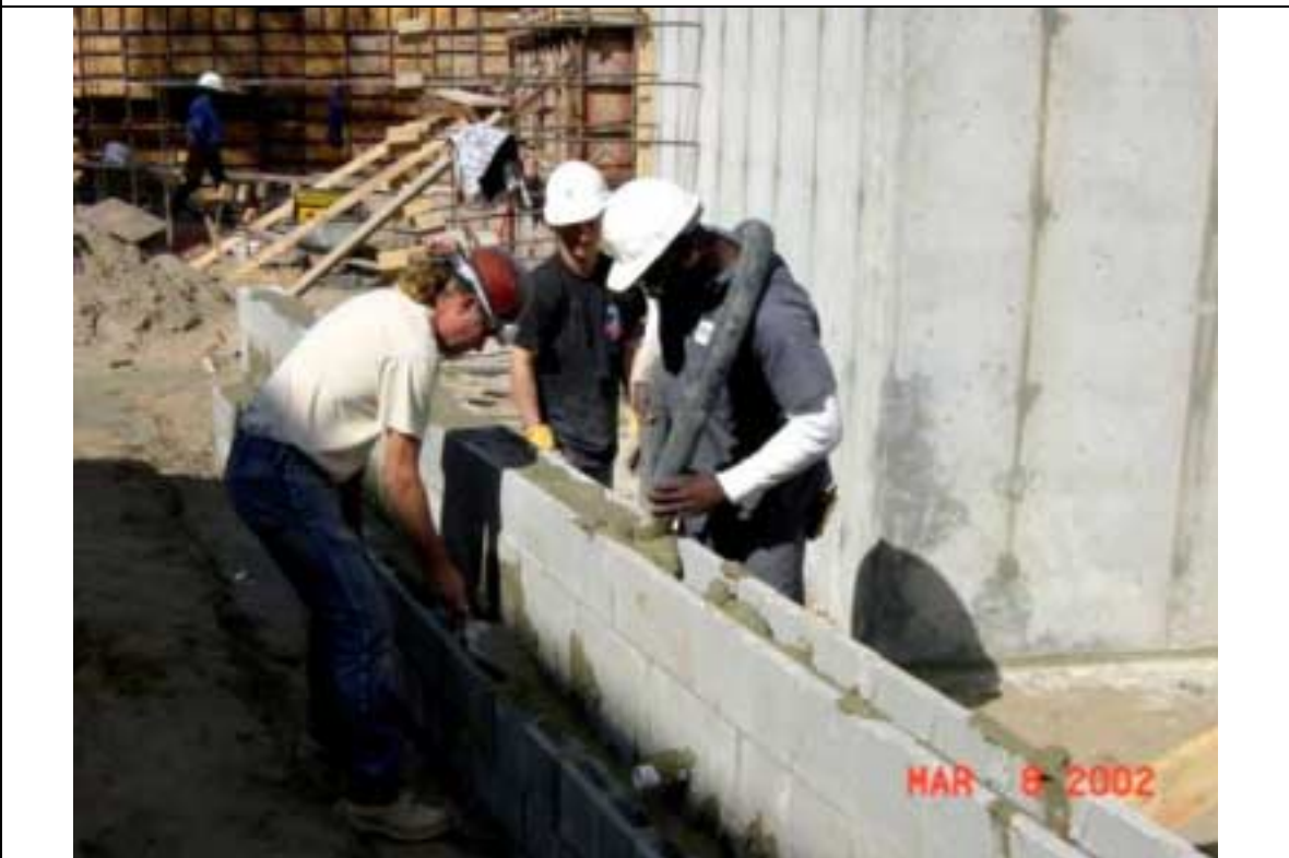
Grouting Serpentine wall.JPG
