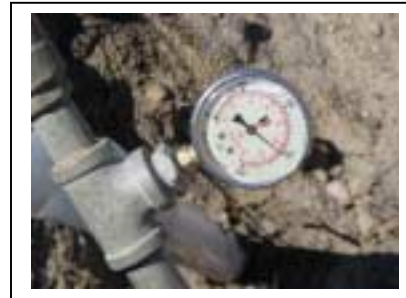
Waterline Pressure Test
