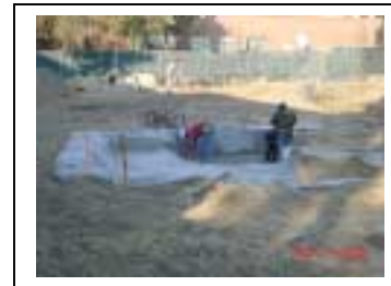
Bentonite Waterproofing at Stormwater Harvesting Vault
