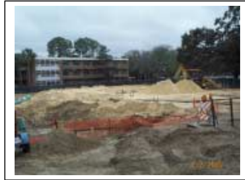
Foundation Work Delayed for Asbestos Abatement
