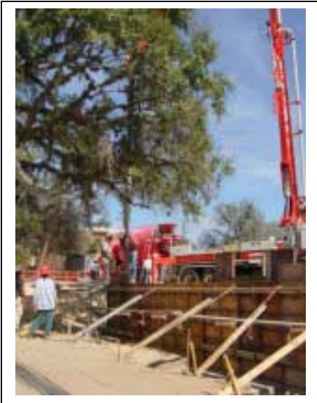
Pouring Cast-In-Place Retaining Walls
