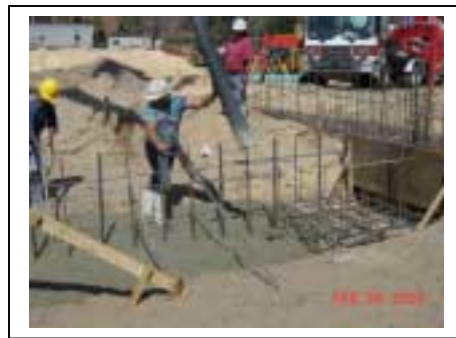
Concrete Foundations
