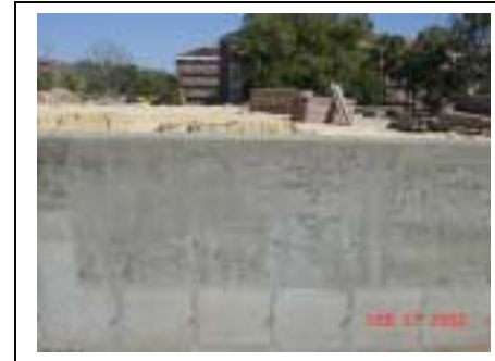
Approved Mock-Up for Exposed Concrete Wall Finish
