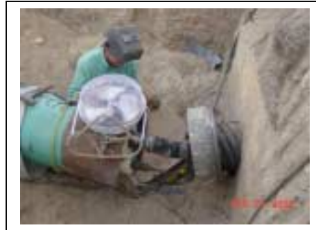
Steam Reroute Tie-In
