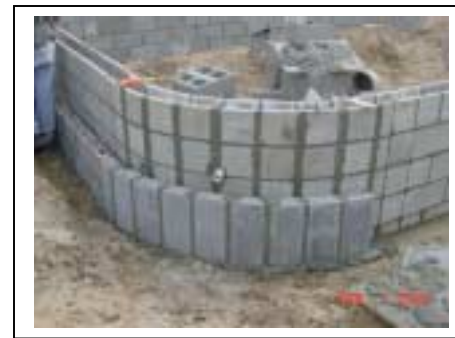
Radius CMU Site Wall along South Property Line
