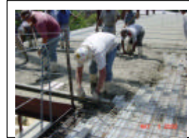
Concrete Pour at 3 rd Floor Elevated Deck
