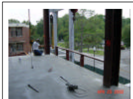
Tube Steel Framing for Perimeter Building Skin
