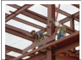
Perimeter closure pieces for metal deck
