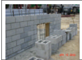
Blockout for Primary Electric at Construction Yard
