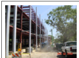
Galvanized Tube Steel for Brick Façade Wall
