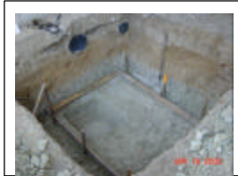
Excavation/Formwork for Steam Pit
