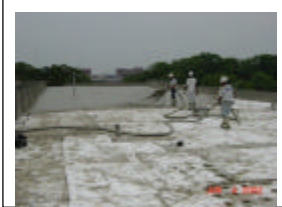
Lightweight Insulating Concrete at Roof
