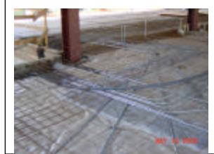
Underground Rough-In & Slab on Grade Prep
