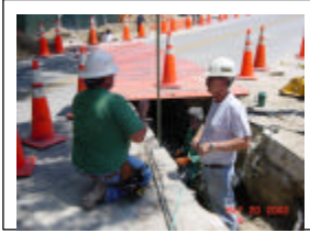
Newell Drive Road Crossing for Steam and Condensate
