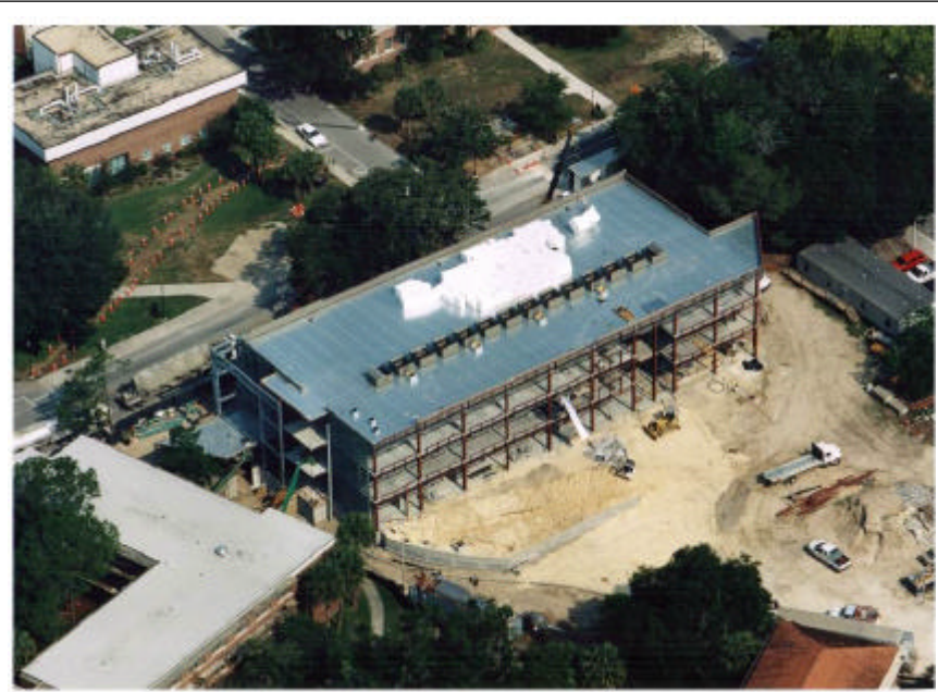
Aerial Photograph Dated June 3, 2002
