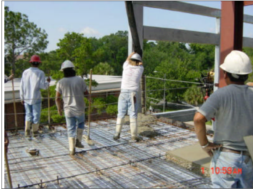
3rd Floor Deck
