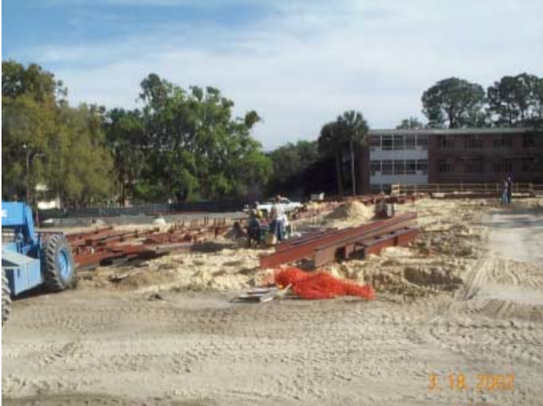
Steel arrival on jobsite 2
