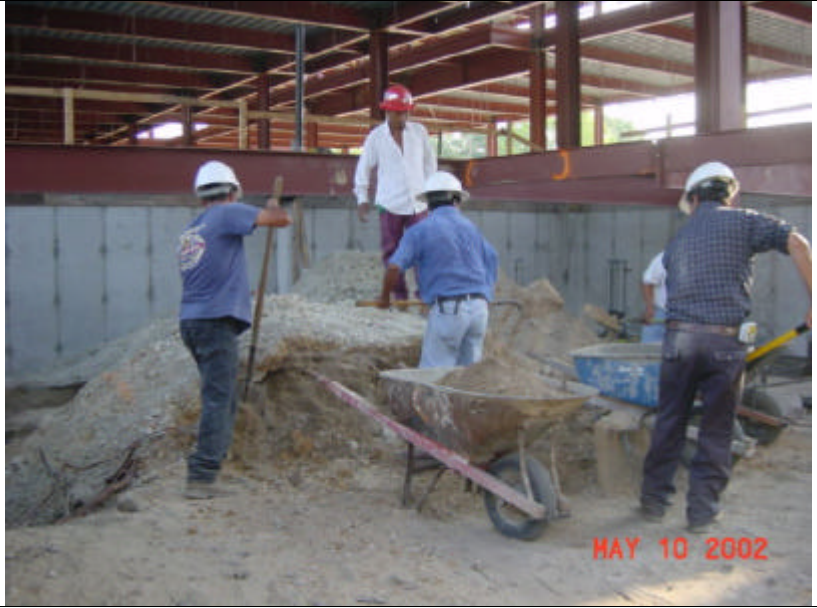
Grading at Mech Room
