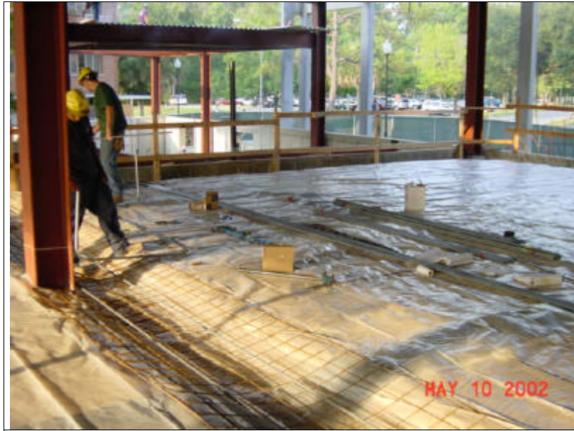
Electrical Rough IN
