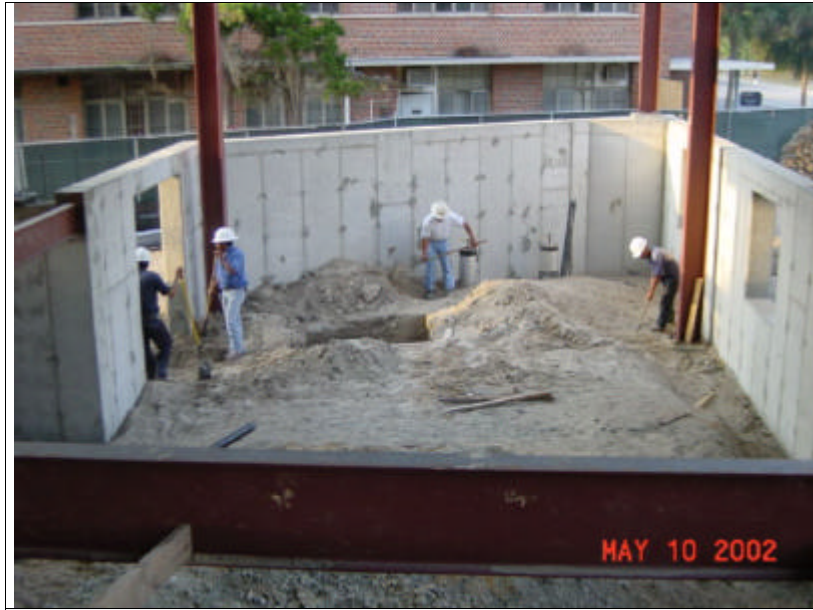
Grading at Mech Room
