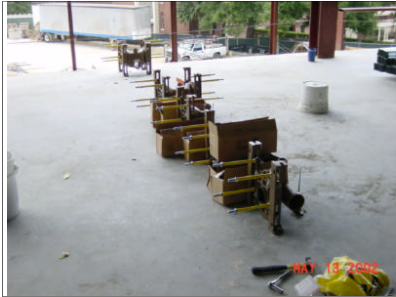
Carriers in place
