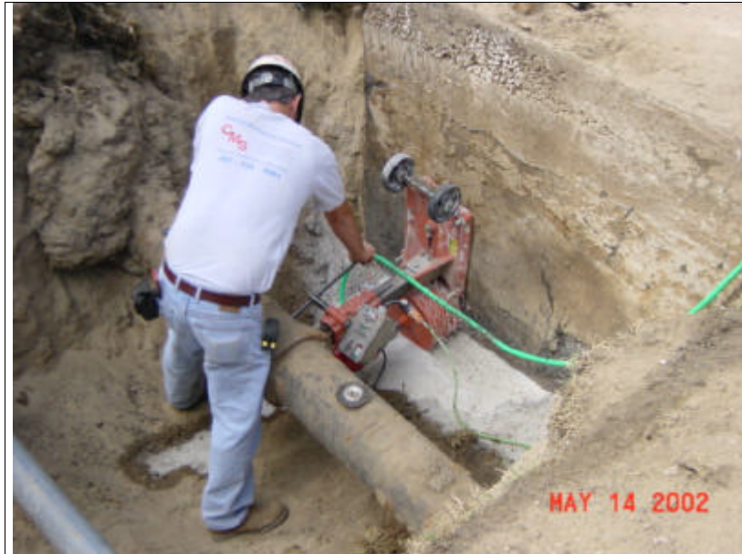
Core Drill Steam Manhole
