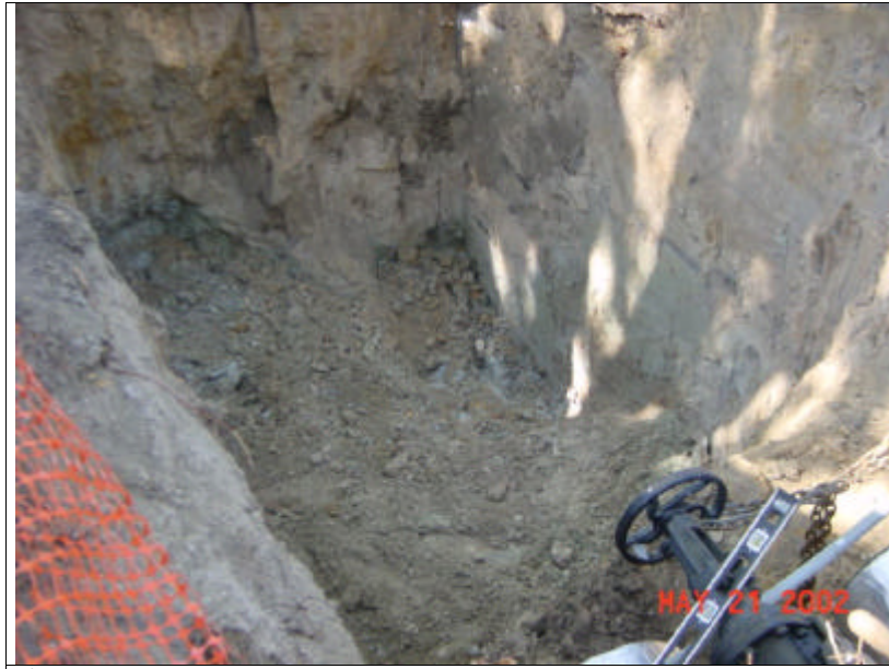
Pit for manhole
