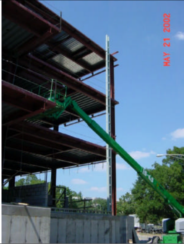
First long studs
