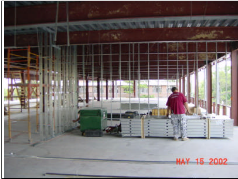
Stud Wall, 2nd floor
