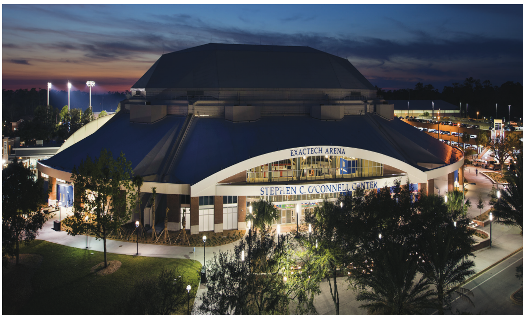
University of Florida Exactech Arena at Stephen C. O'Connell Center, Gainesville, Florida
